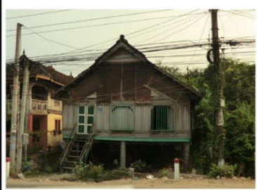
the concrete pillars
