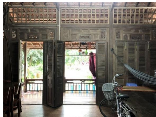
Figure 24 Wooden doors with louvres in a three-compartment house.
