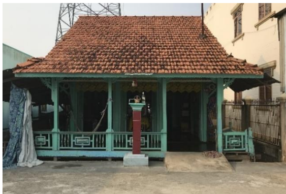
Figure 23 Basic module of three-compartment house with veranda at the front.
